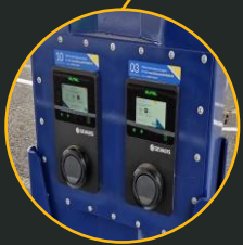
12 x 22kW AC Charge Points
